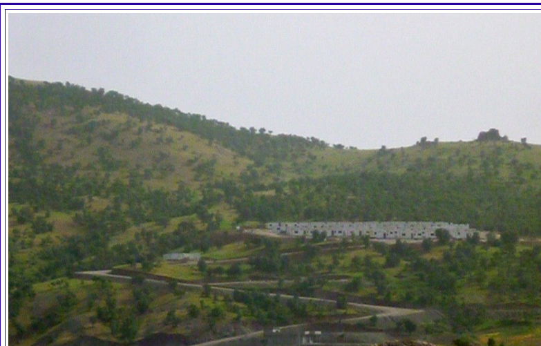
New IDP camp under construction few kilometers from Gojar camp
