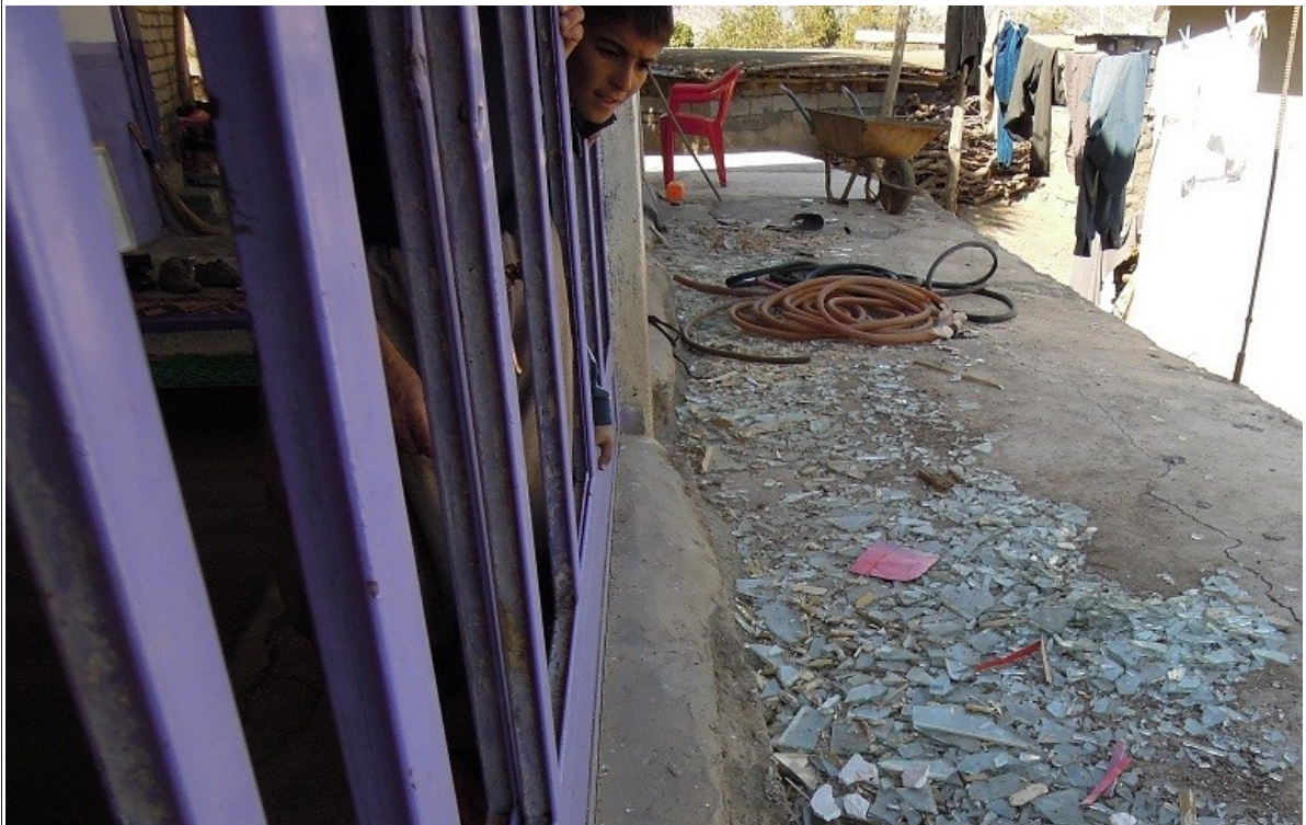
Shattered windows by shelling - Sunnah village
