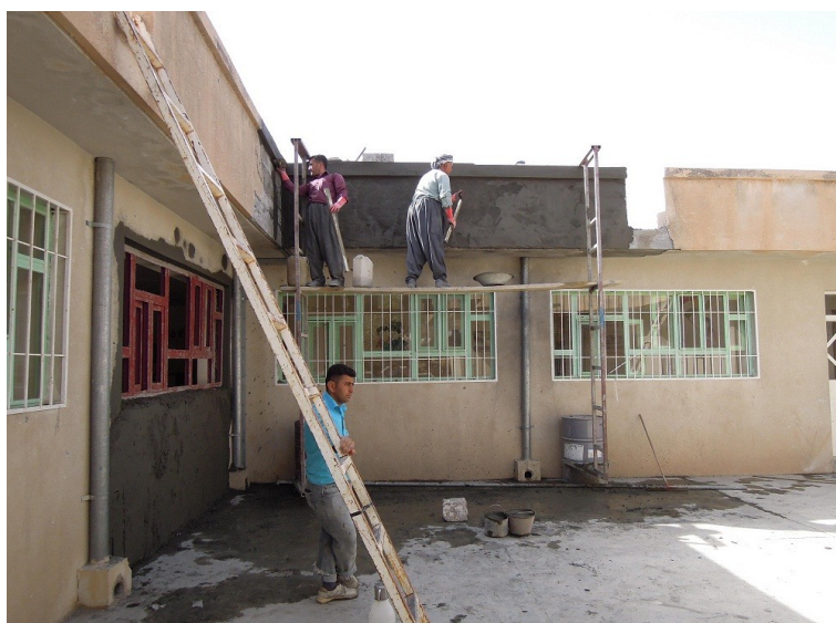
Sunnah school under repair from the damages
