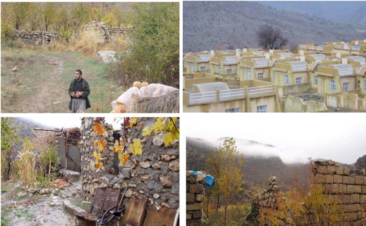
Abandoned village: Trwanish, Kani Mase, Nov 2008. Destroyed building on lower left is a school.
